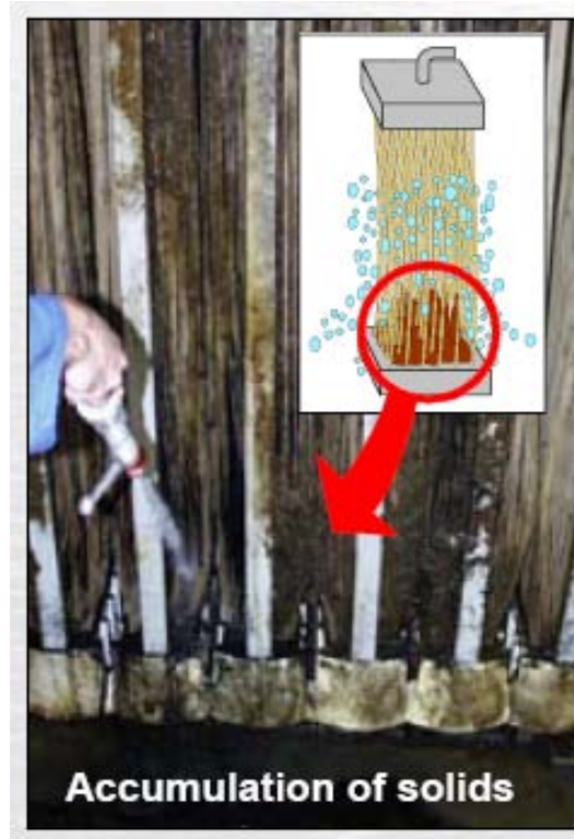
Membrane fouling at bottom
